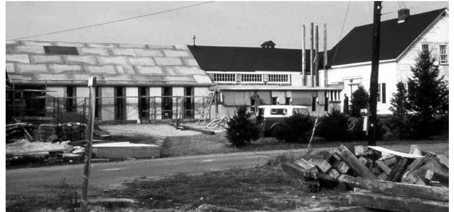
Stone Chapel under construction, 1964
