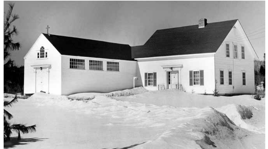
Renovated chapel and monastery, around 1953
