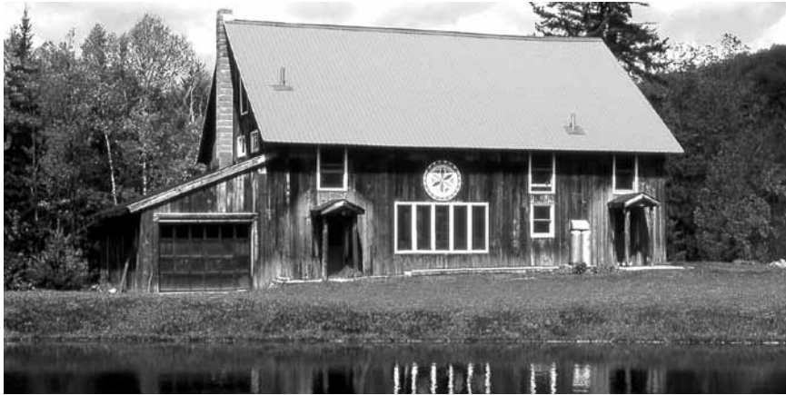
Extension Community House (East Family House), 1977
