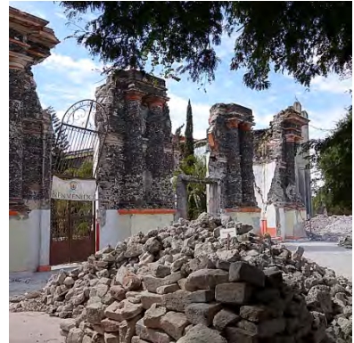
Jojutla - destroyed buildings.
